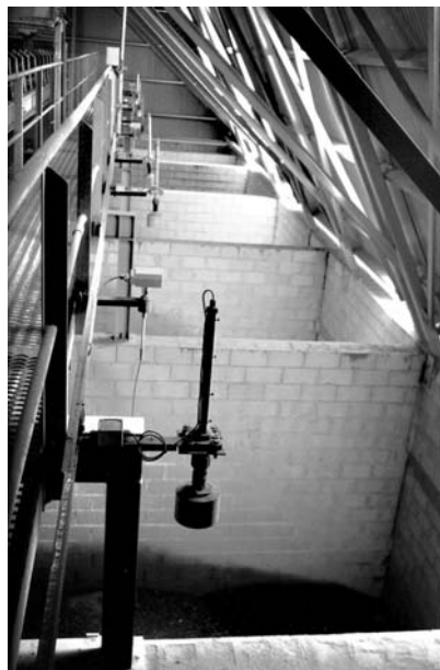
Measurement of sand, gravel etc. in open bins
