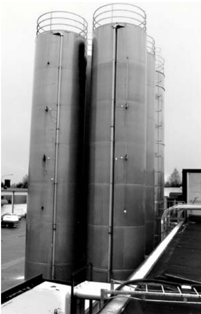
Measurement of plastic pellets in 16 m silos
